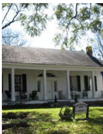
Square Columns in Greek Revival Style
