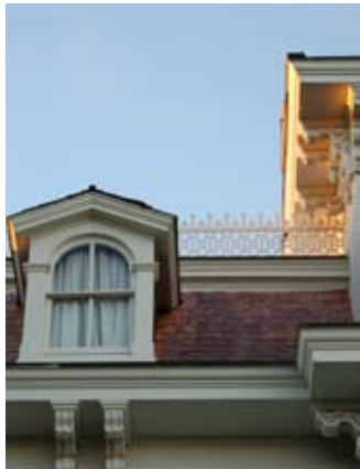
Dormer Window with a dormer head
